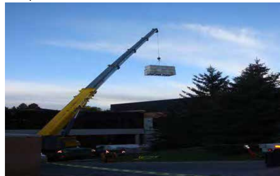
Chiller Replacement Project
